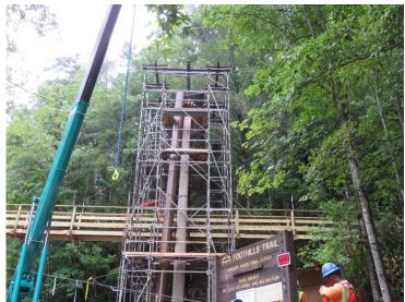
bridge! After studying all angles of this enormous task, they also decided that the best material for the longest life of the bridge was fiberglass. This would be much lighter to transport to the site, but also would be very long-lasting. Thus, the entire supporting structures at either end, as well as the tread of the bridge, are made of fiberglass. The handrails and cross supports are the only wooden portions. The supporting cables are the only original materials.
